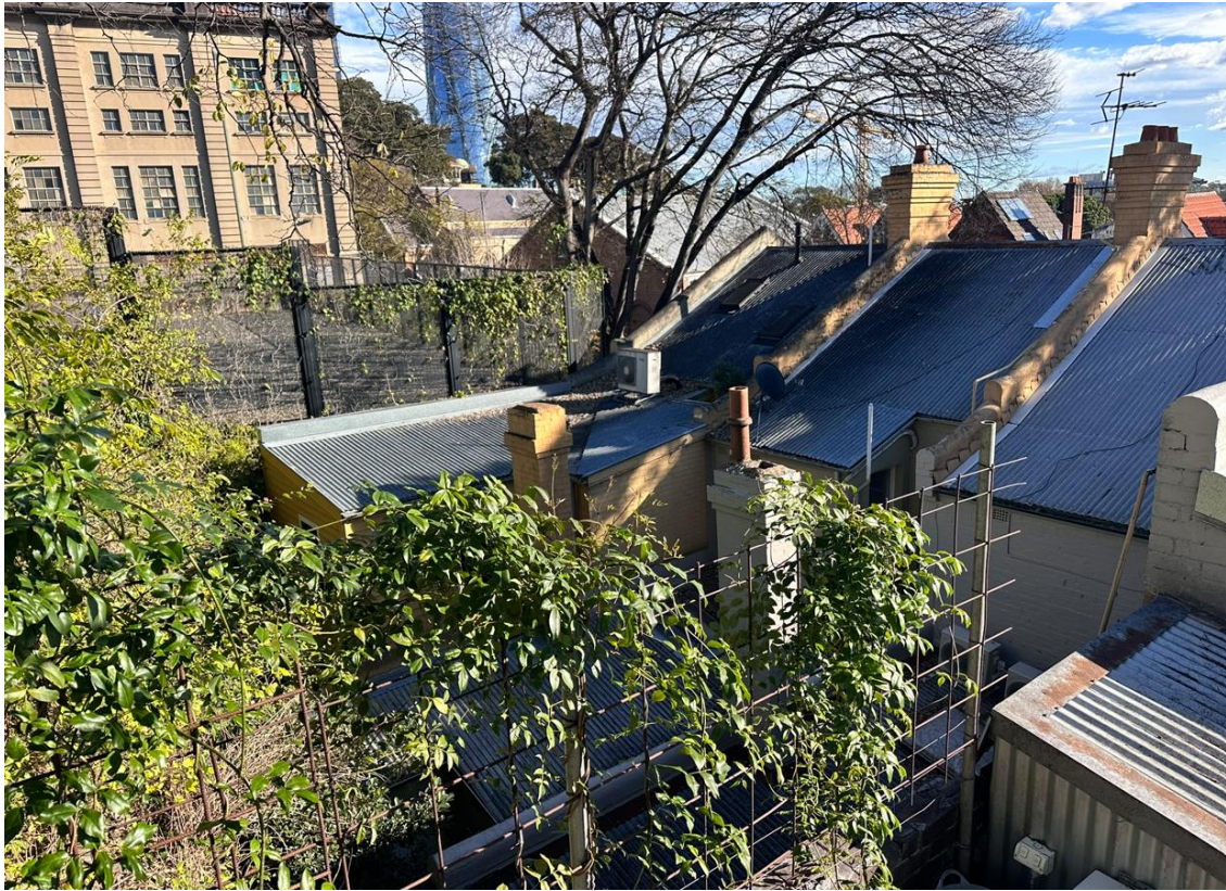
Figure 5: View to the rear of 18 to 22 Trinity Avenue
